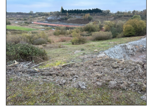
View of the slip viewed from the V-cut.
