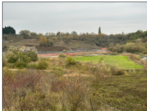
View of the works from the extension track.
