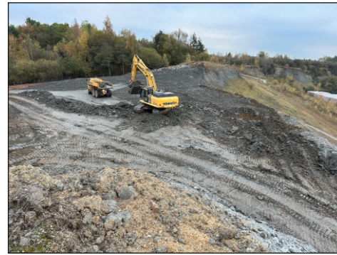
Digging out the V-cut, looking towards the brickwork viewing area.
