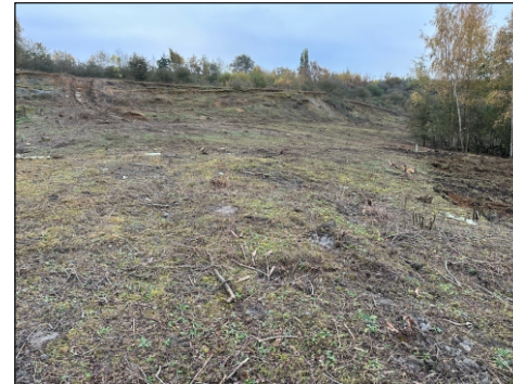
Majority of the upper slope is cleared. Trees were also cleared last week.
