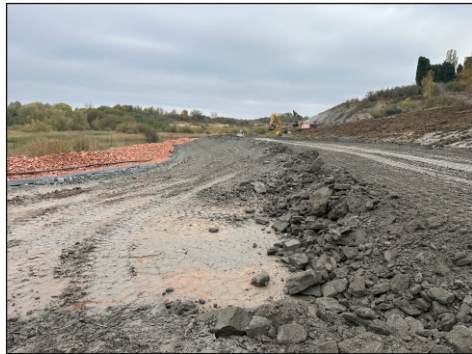
Putting in the clay lifts. The visible bricks area against the water.
