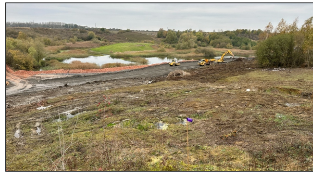
Panorama of the works proceeding.
